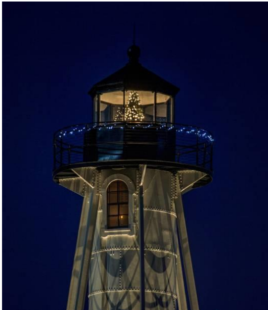
Boca Grande Lighthouse, Florida
